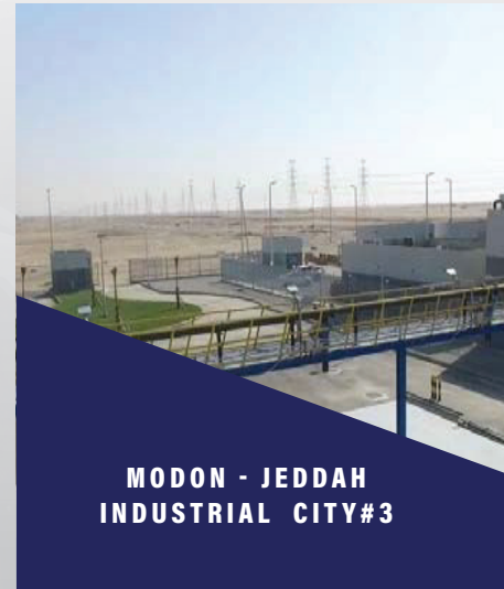
MODON - JEDDAH INDUSTRIAL CITY#3
