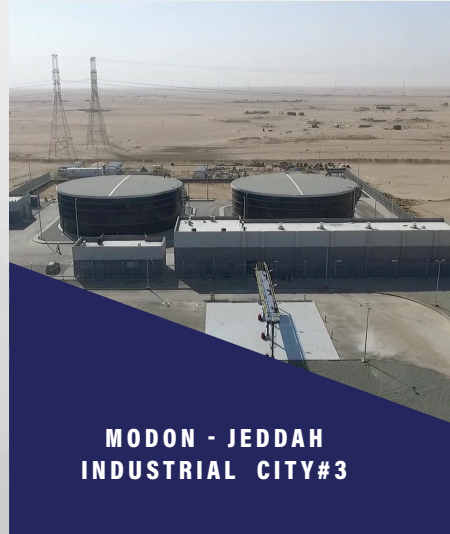
10,000 m3 Water Treatment Plant with GLS Tanks & Pumping Station
